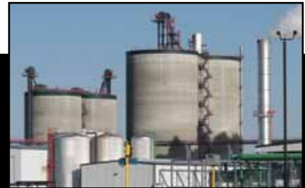
Nebraska Ethanol Plant
