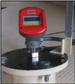
Actual installation on rice bin.
